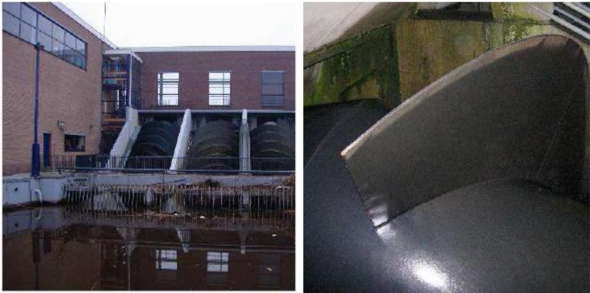
Figure 2.1 Example of a conventional screw pump with on the right side a detail of the winding
